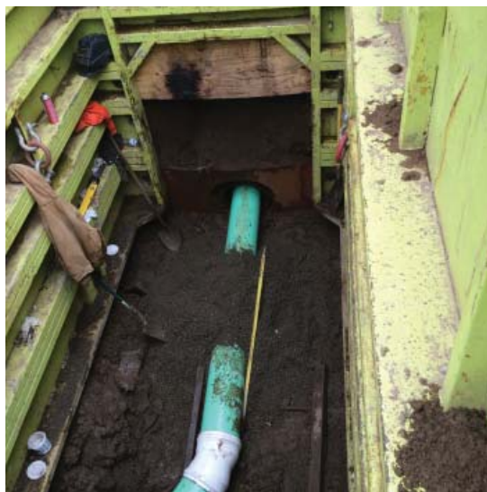
A 170-foot-long bore placed a 20-inch steel casing along the alignment.
