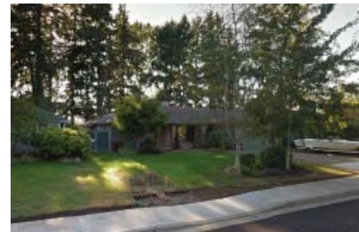
Home built over storm drain prior to second story addition.
